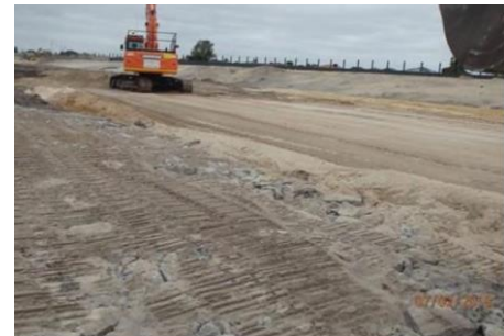
Figure 3: 300mm lift track rolled 4 passes.
