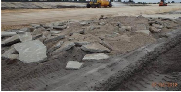
Figure 1: Material broken down in demolition process and carted to fill area.
